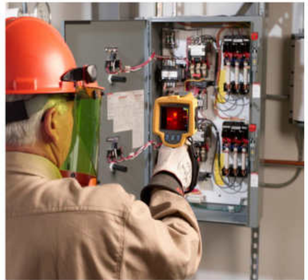
Fig III Image capturing with IR camera
